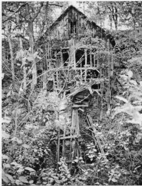
Thwing Mill in 1985, prior to reconstruction
